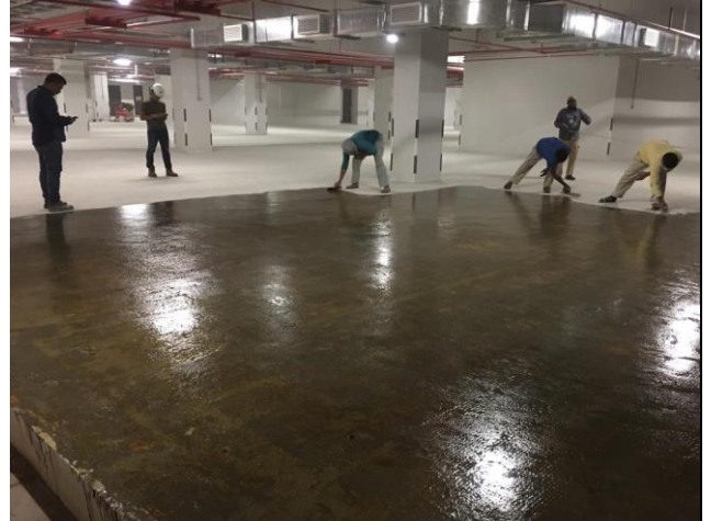
Aras Besmen – Moisture barrier installation
