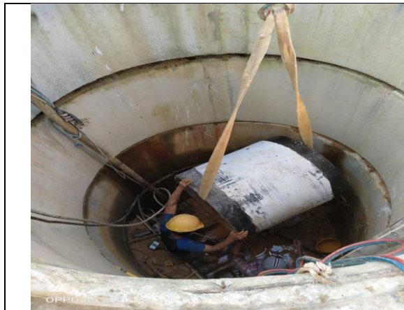
MH6-MH8 – Manshield pipe sleeve jacking
