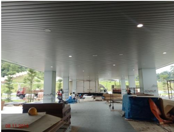
Blok MP – Covered walkway / porch
