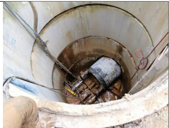
MH6-MH8 – Manshield pipe sleeve jacking
