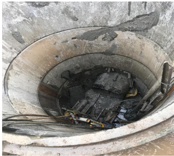
MH5 –MH5S – MH6s – Manshield pipe sleeve jacking
