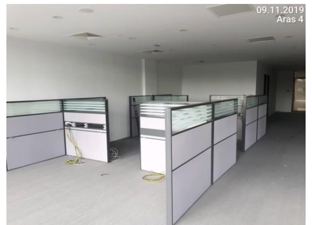
Aras 4 – Pemasangan workstation
