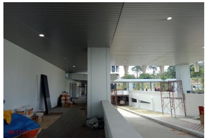
Blok MP – ramp to besmen
