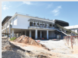
Pembinaan bangunan stesen Construction of station building
