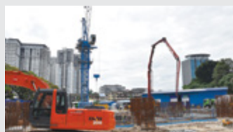
Pembinaan raft foundation Construction of raft foundation
