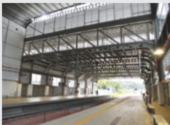
Pembinaan Platform 1 & 2 Construction of Platform 1 & 2
