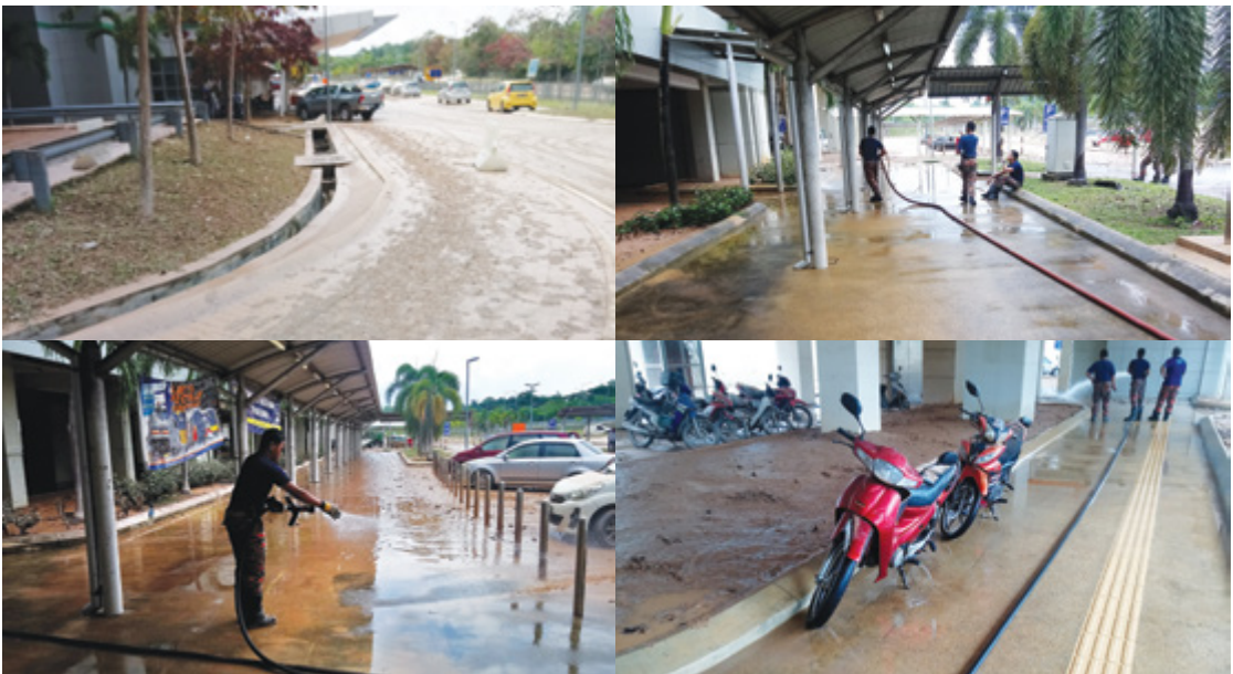
Gambar 25: Kejadian banjir kilat di Stesen Keretapi Sungai Gadut, Negeri Sembilan pada Oktober 2019 Picture 25: Flash floods at Sungai Gadut Railway Station, Negeri Sembilan in October 2019
