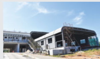
Pemasangan Portal Frame Installation of Portal Frame
